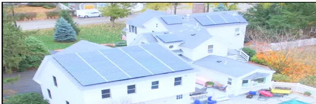
Figure (3) Installing Solar on a Roof
